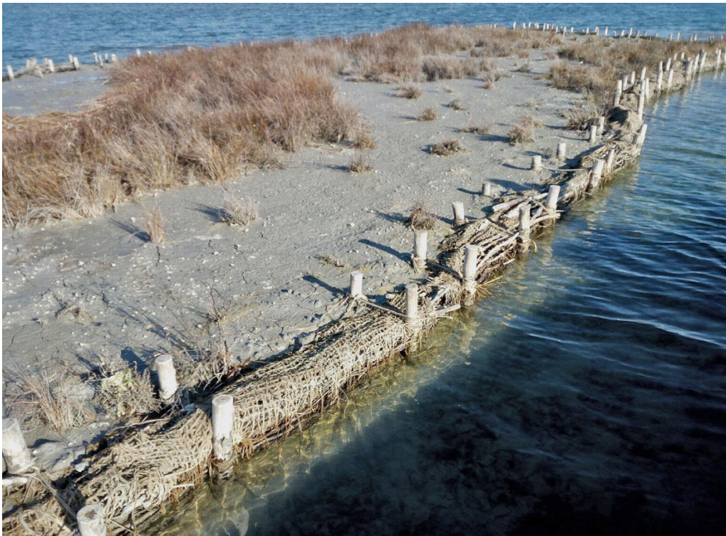
Figure 8: Nature-based solution in live willow; northern lagoon. (prof Barause marine conservations principles and applications class)
