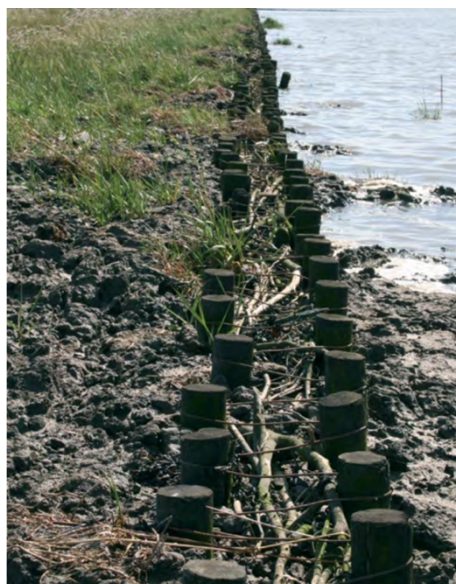
Figure 4: Brushwoow groynes to protect salt marshes against lateral erosion (August
