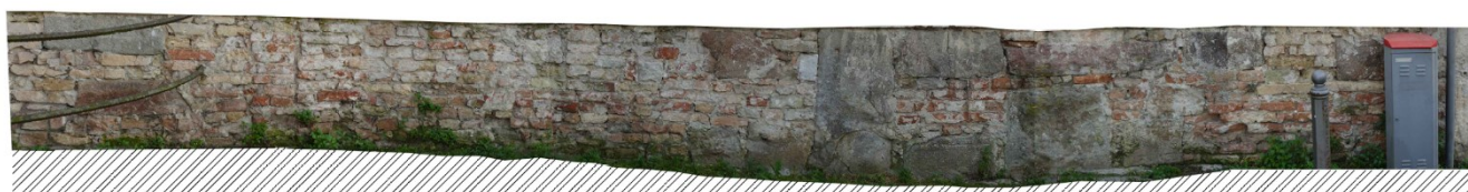
Figure 27: Orthophoto of North wall.
