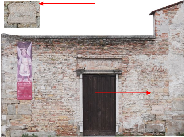
Figure 1: Reused materials visible on the North wall of S. Michele.
