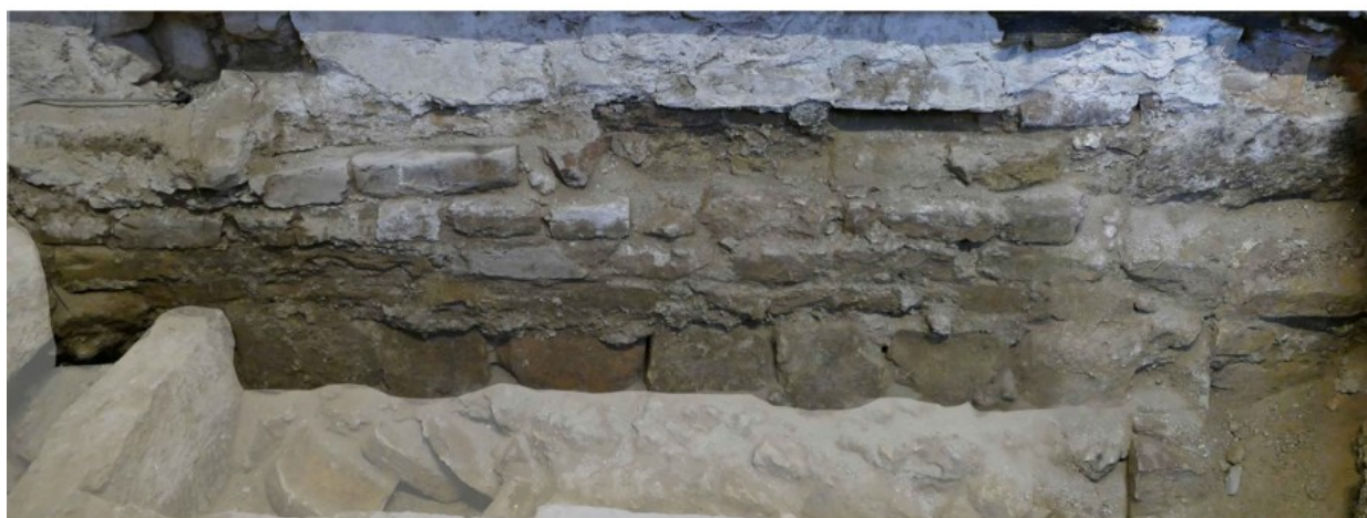
Figure 35: Orthophoto of the Northern excavation wall
