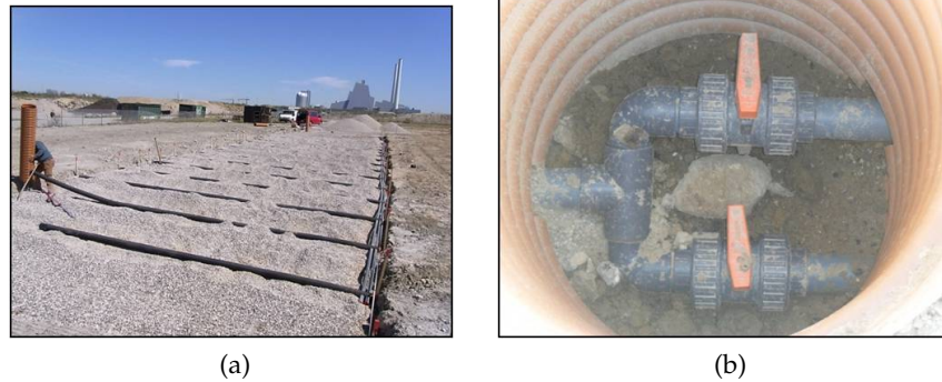
Figure 10: (a): Front view of the biocover distribution layer, (b): Valves sites at biofilter distribution system inlet.
