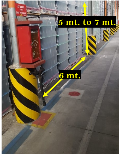
Figure 19: Width between columns, 6 mt., and height 5 mt. in the temporary warehouse, 7 mt in the definitive warehouse
