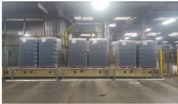
Figure 13: Picking stations for pallet pairs from the roller conveyor in the receiving area
