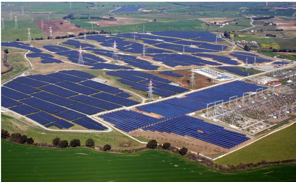
Figure 51 View of the Montalto di Castro Power Plants
