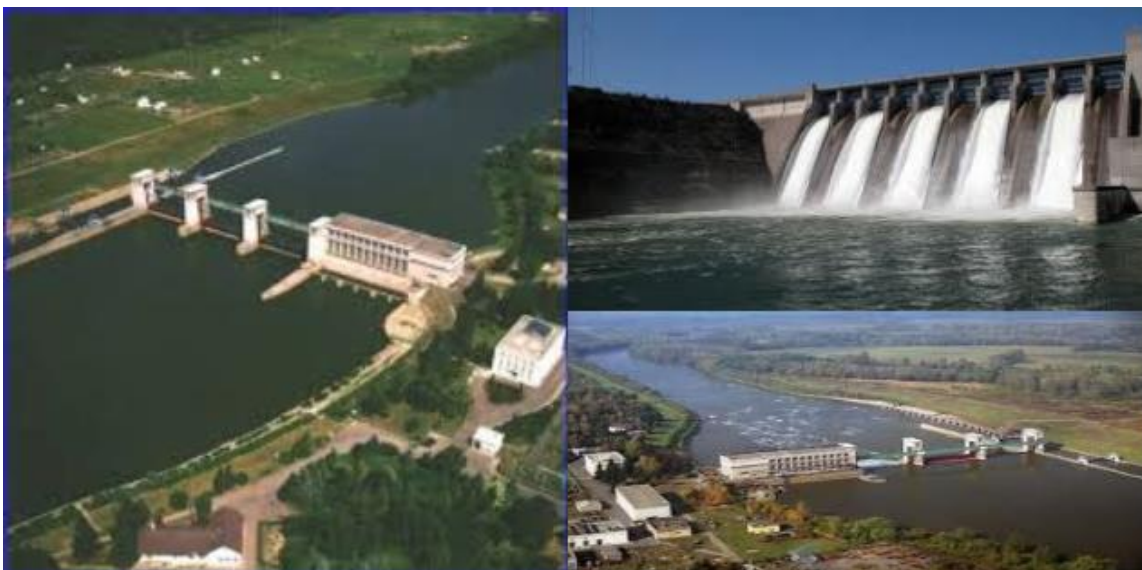
Figure 26 Tiszalök hydropower plant
