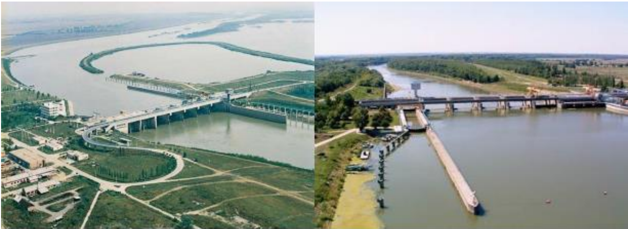
Figure 29 Kiskore hydropower plant
