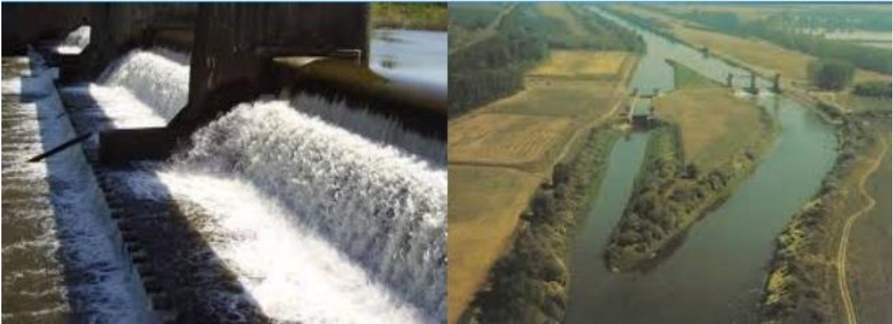
Figure 27 Kenyer hydropower plant
