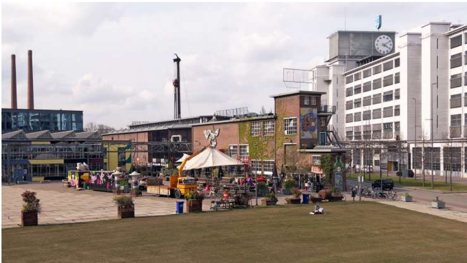
Fig.86 View of the High-voltage building. (Source: personal elaboration)
