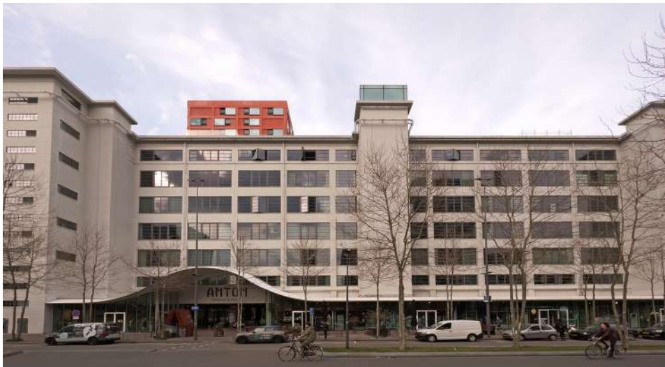
Fig.87 View of the Anton, the westernmost building. (Source: personal elaboration)
