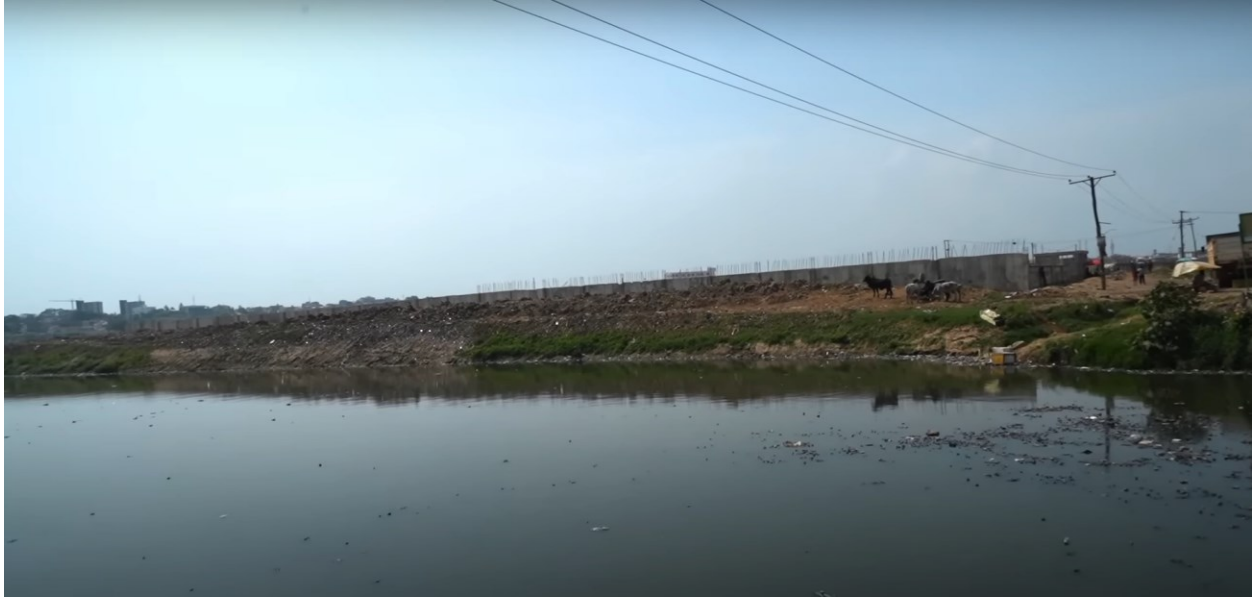
Figure 7 picture of the wall erected by the government copyright https://www.youtube.com/watch?v=sTio_0rwR1s&t=502s
