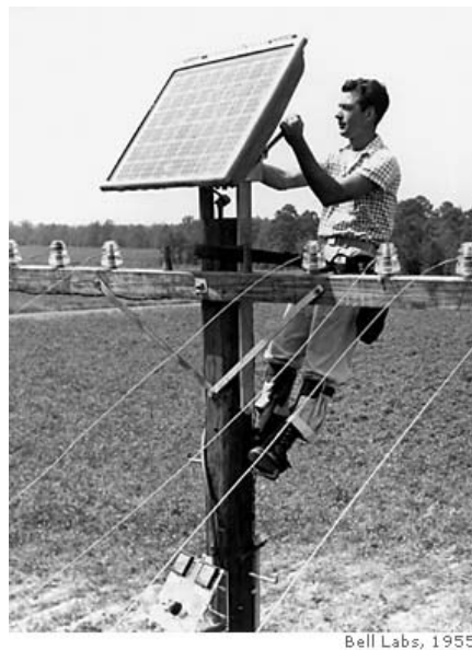
Figure 1.1. Photograph of original Bell Solar Battery installation in 1955. Source: https://www.bellsystemmemorial.com/belllabs_photovoltatics.html .
