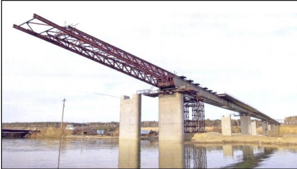
**Figure 1.5.** Incremental launching of a plate girder
