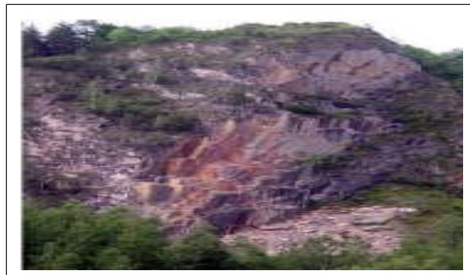
Figure 1.9. Block topple in limestone, Czech Republic.
