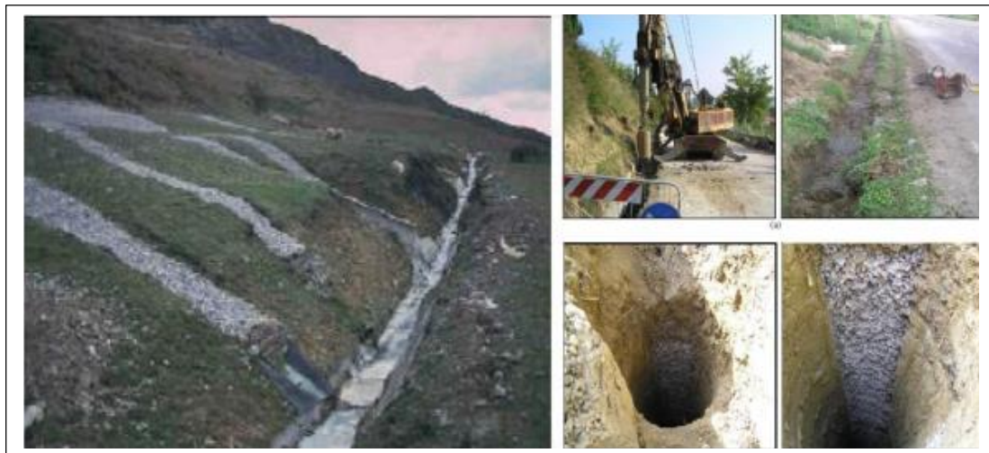
Figure 1.23. Examples of a shallow and deep drainage trenches (Van Impe, 1989)
