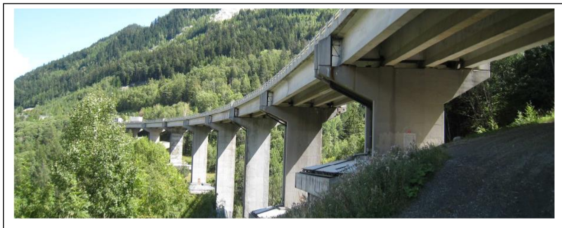
Figure 3.2. Charmaix Bridge, lateral view.
