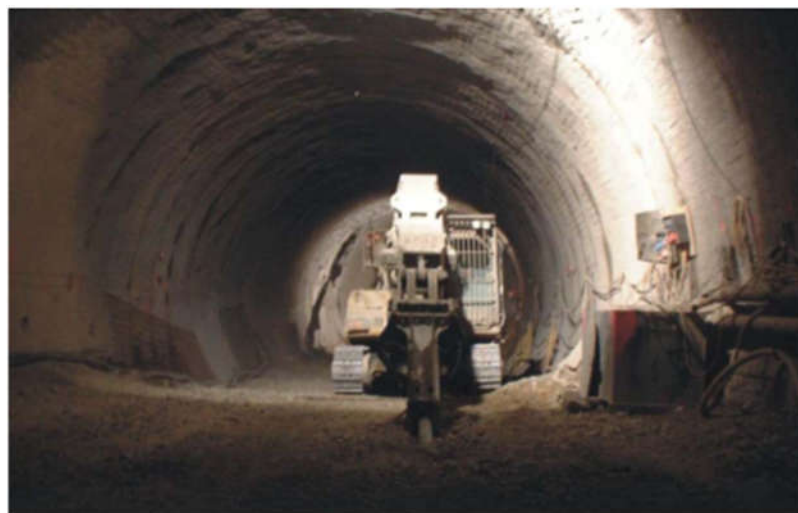
Figure 3.5. Construction of the Steinhaldenfeld Tunnel(Möller et al., 2004).
