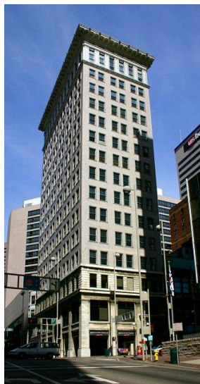
Figure 1.4. Ingalls Building (Photo by Rick Dikeman)
