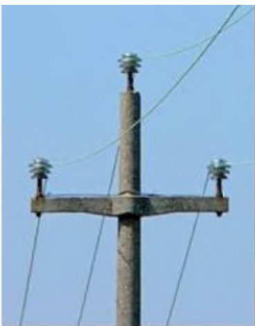
Fig. 1.7a. Simple supporting insulator
