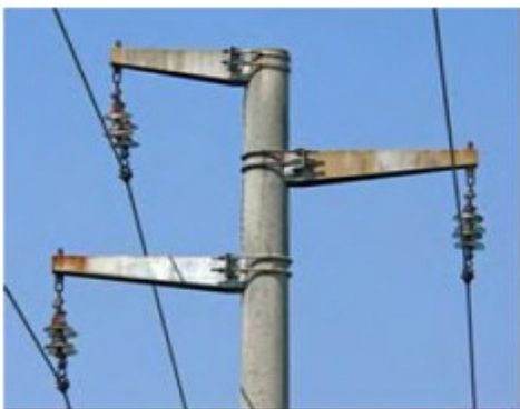
Fig. 1.9a. Suspended insulator
