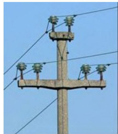
Fig. 1.7b. Double supporting insulator
