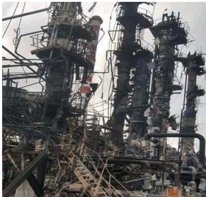
Figure 1.27. Damaged SONARA structure (crtv.cm, 2022)
