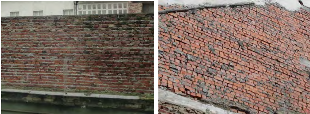
Fig. 1.9.2: Uprising masonry (US 100 and US 85)
