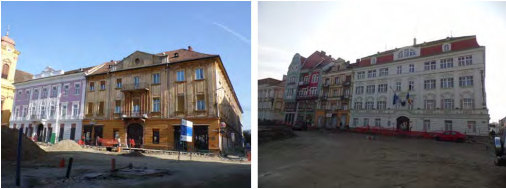
Fig. 1.8.7: Widely holed facades(Blocks C9 and C16)
