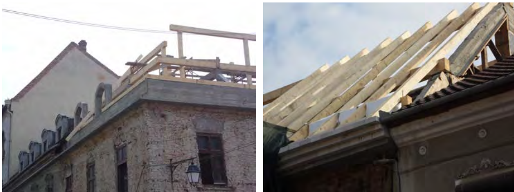
Fig. 1.9.20: Non –thrusting mixed roof examples (US 82)
