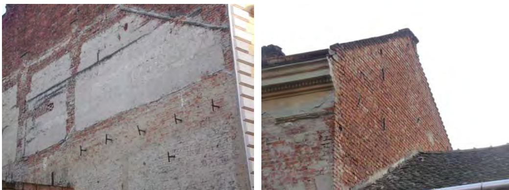
Fig. 1.10.3: Tie rods examples(US 79 and US 237)
