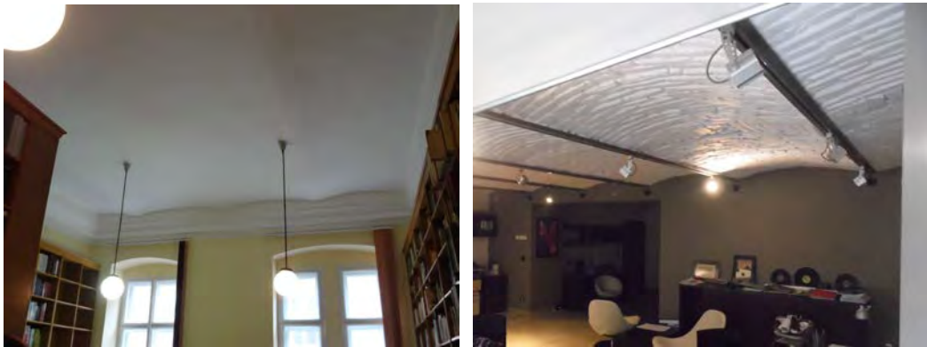
Fig. 1.9.15: Iron beams and little brick vaults examples(US 100 and US 3)
