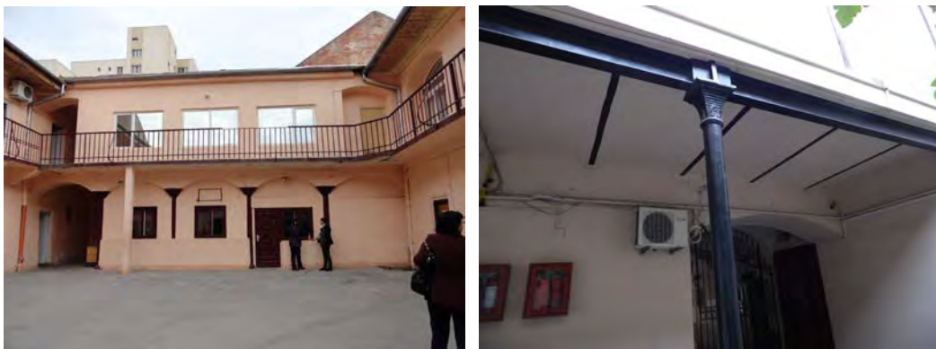
Fig. 1.9.5: Solid metal columns(US 8 and US 28)
