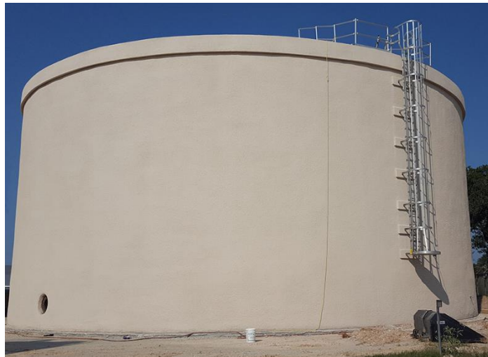
Figure 1.19. Prestressed storage tank (Bald et al., 1997).
