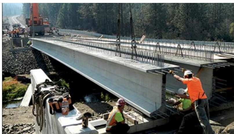
Figure 1.7. Prestressed concrete girder(Boukendakdji et al., 2017).
