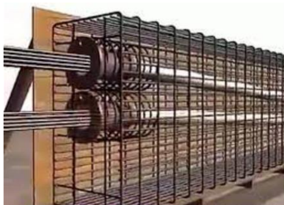
Figure 1.5. Non prestressed steel reinforcement (Bymaster et al., 2015).
