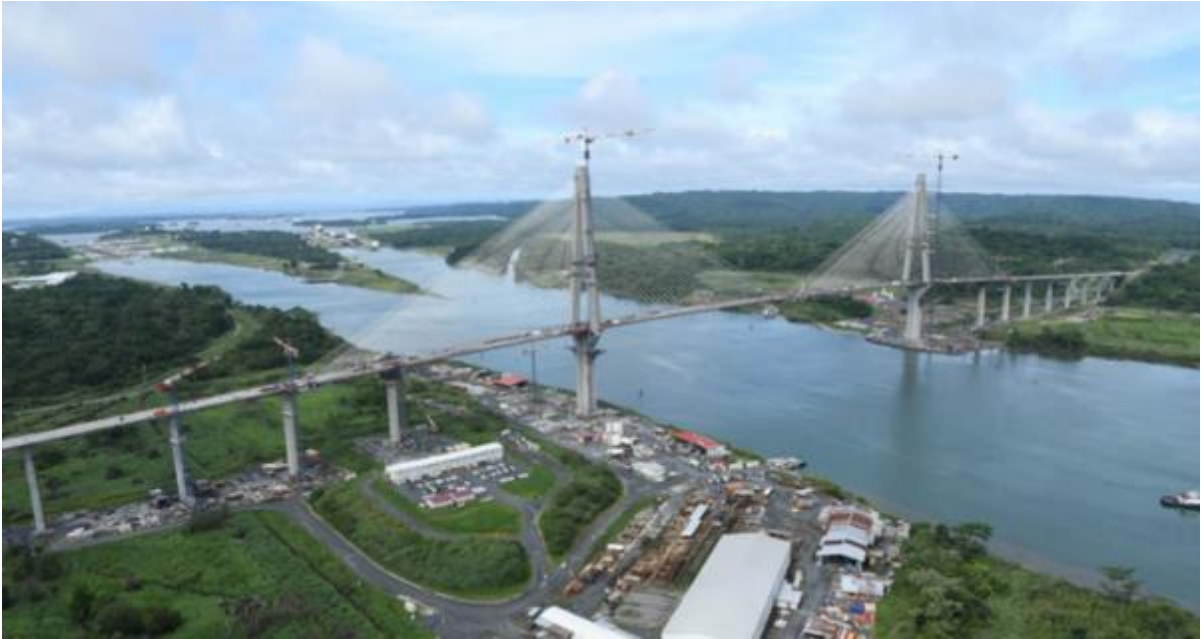
Figure 1.35. The Panama Atlantic bridge(Craig, 2018).
