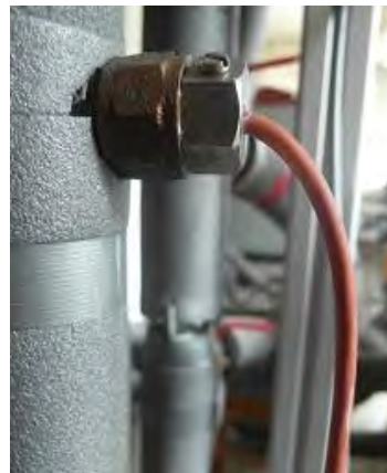
Fig.3.3.2 - Pt 100 thermal sensor
