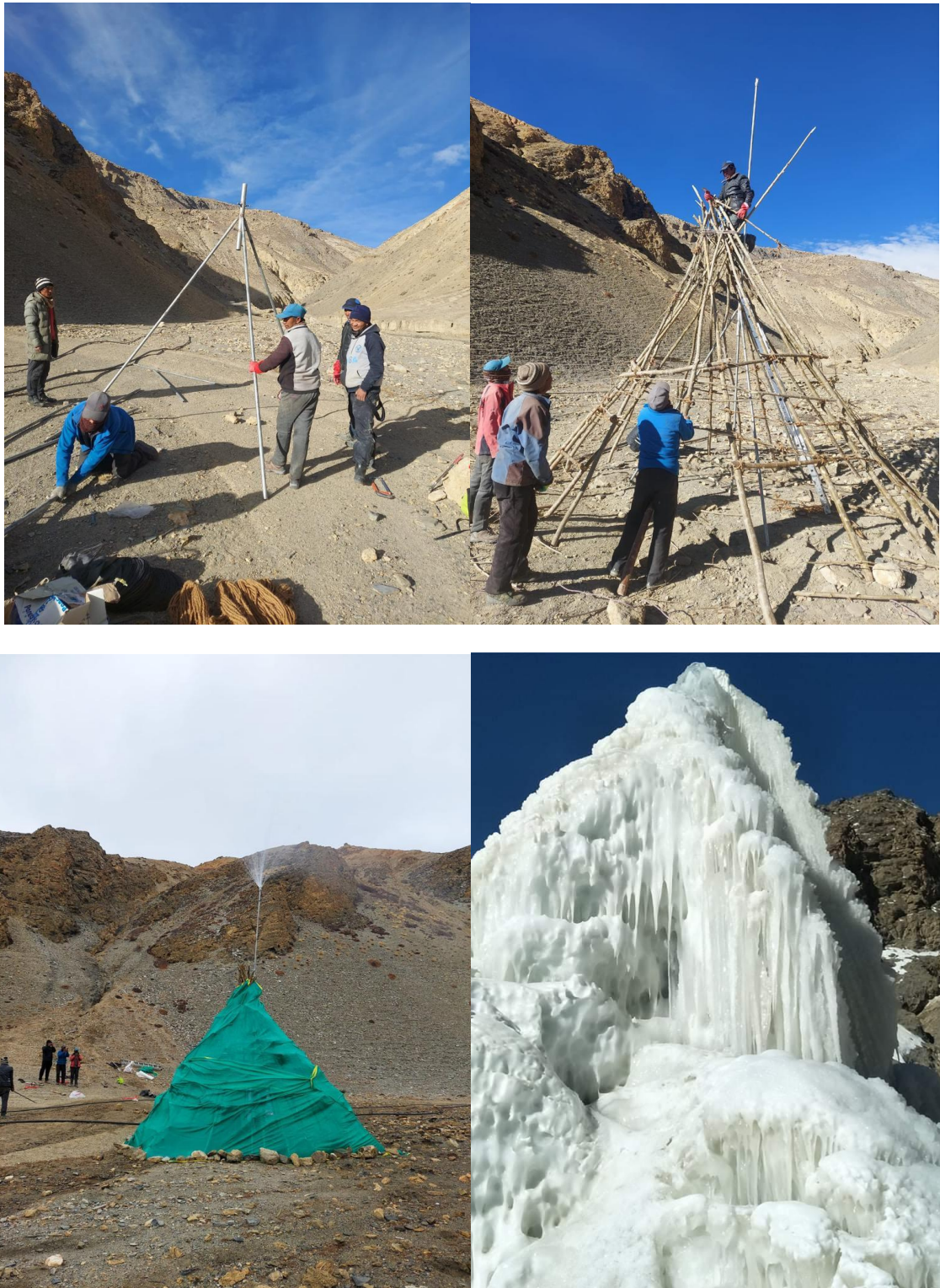
Picture 5. Different phases of construction of the ice stupa (Videh Foundation, 2022)
