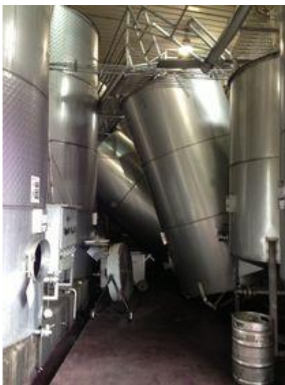
Fig 1.5: Steel tanks collapse in a Napa winery.
