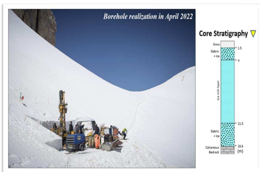
Figure 54. Borehole realization after geophysical investigations in Calderone glacieret (April 2022)
