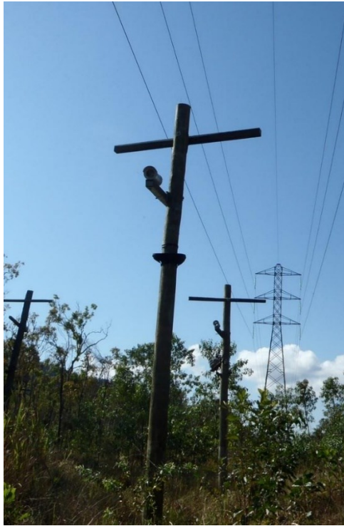
Figure 4.6: Example of glider pole. Image from Glider Poles Successful in Helping Animals Jump across Australian Highways | News.Com.Au — Australia's Leading News Site.
