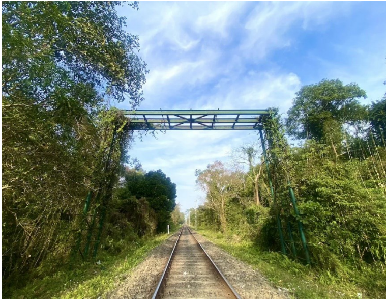
Figure 4.5: Example of semi-artificial canopy bridge. Image from NFR To Install Canopy Bridges in Hollongapar Gibbon Sanctuary - The Hills Times.
