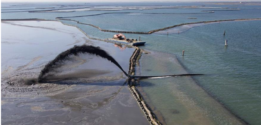
Fig. 16, Sediment drainage for construction of artificial salt marshes.
