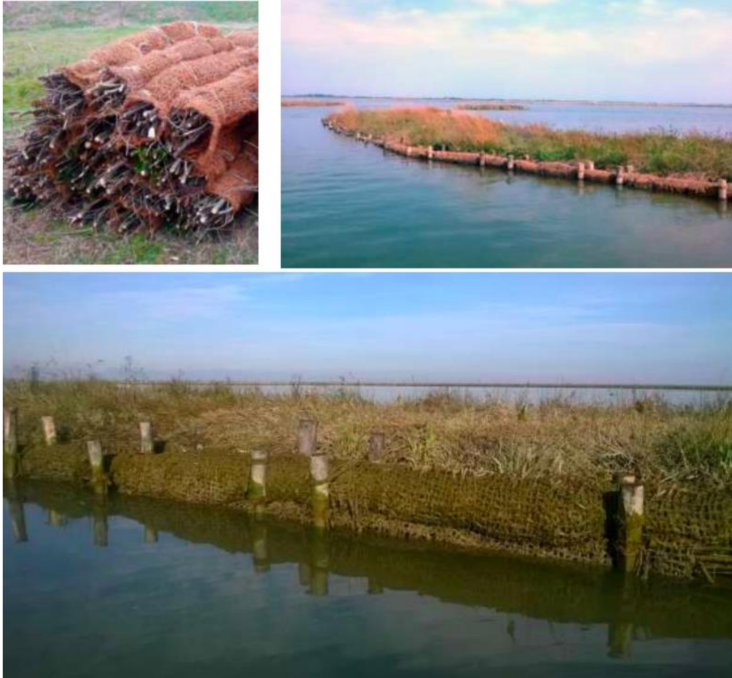
Fig. 19, Fascines produced locally -upper left- and then placed to protect salt marsh edges -upper right and bottom- (Barausse et al. , 2015).
