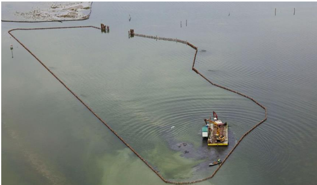
Fig. 15b, Construction of artificial salt marshes near Valle di Brenta, aerial view, southern Venice lagoon, 26-08-2014
