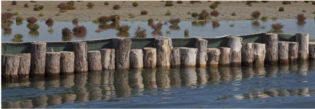
Fig.15a, Poles boundaries during the construction of artificial salt marshes, Venice Lagoon, 19-09-2013
