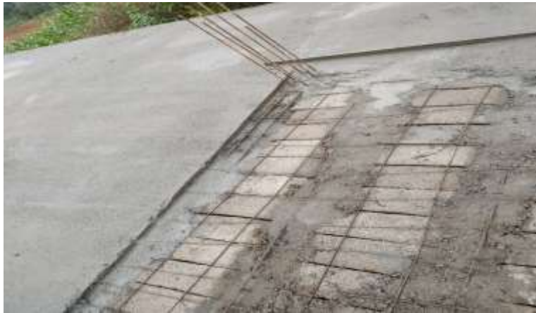
Figure 1.5. Hollow block slab
