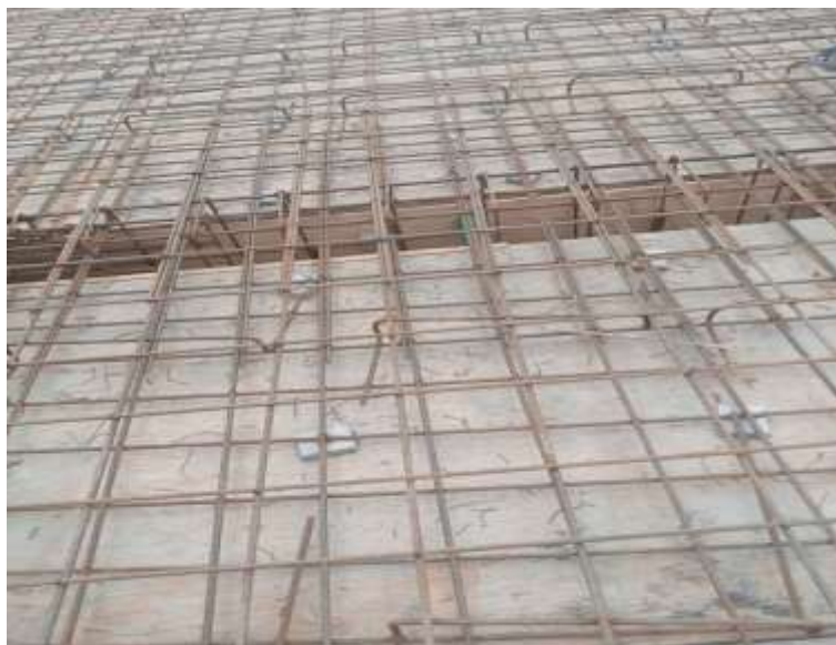
Figure 1.2. Conventional two-way slab (Nlongkak, Yaounde)
