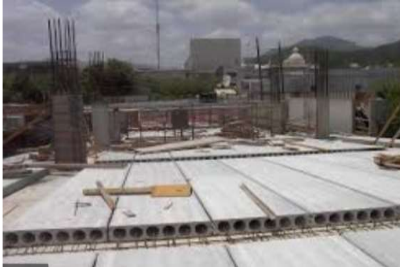
Figure 1.3. Hollow core slabs (www.civilread.cm)
