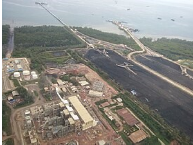
Picture 3. Aerial view of Tanjung Bara. Source: https://en.wikipedia.org/wiki/Tanjung_Bara
