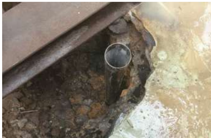
Figure 4.39. PVC – grout casing for injection hole (from data project)
