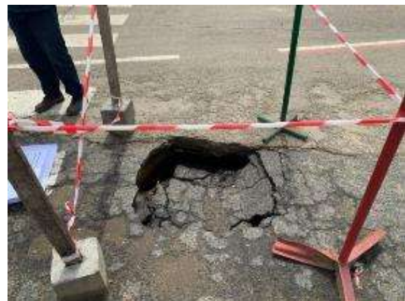
Figure 4.6. Ground collapse inspection (L) close to a building (R) on a paved road
