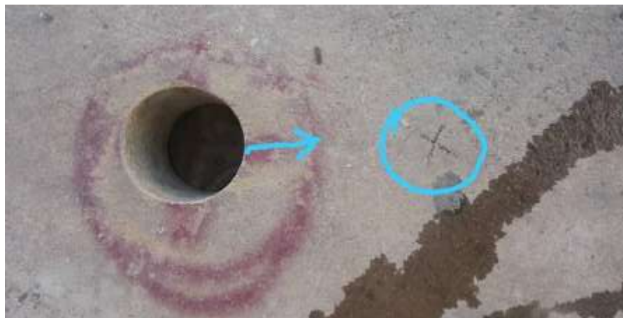
Figure 4.41. Slab coring before injecting (from project data)
