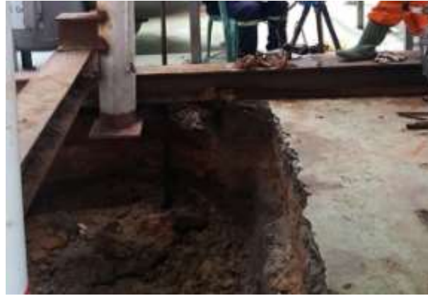
Figure 4.5. Excavated foundation below a storage tank
