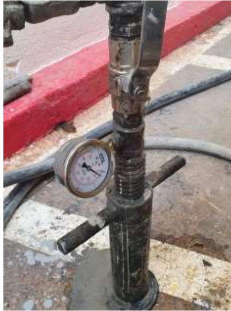
Figure 4.42. Single headers while grouting a hole (from project data)
