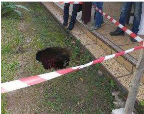
Figure 4.6. Ground collapse inspection (L) close to a building (R) on a paved road
