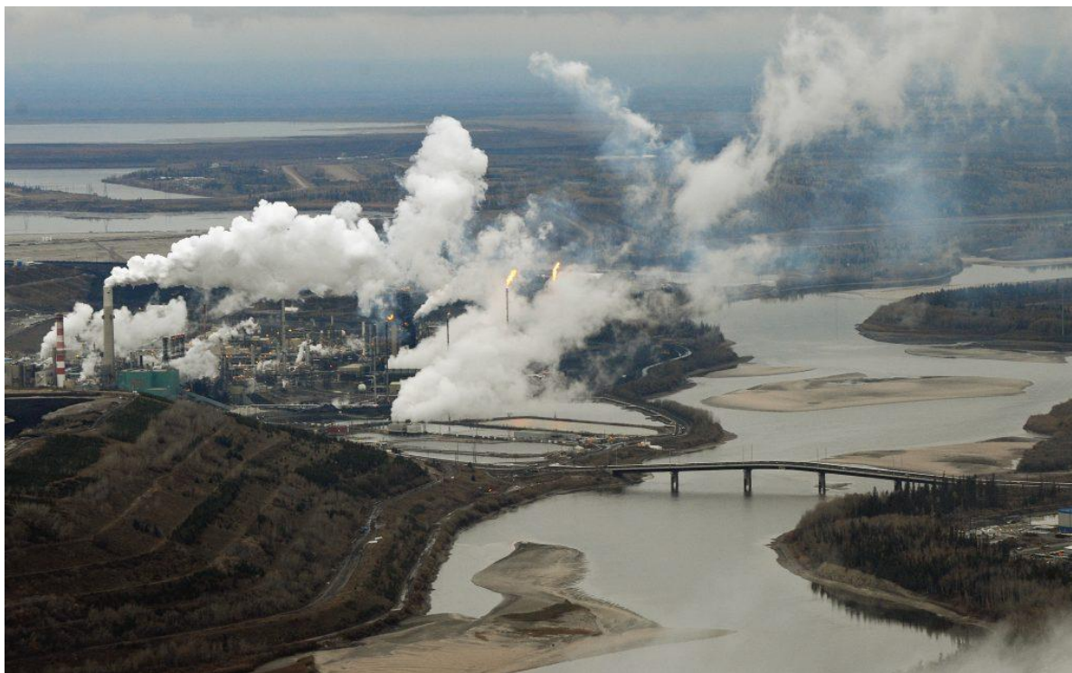
Figure 14: Suncor tar sands facility with tailings ponds
