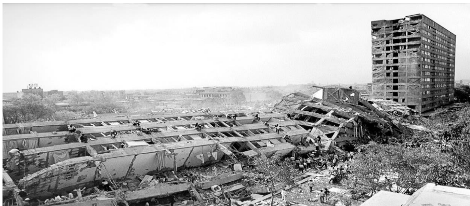
Figure 1. 12. Heavily damaged buildings in Mexico City, 1985. (Image by David Tenenbaum)
