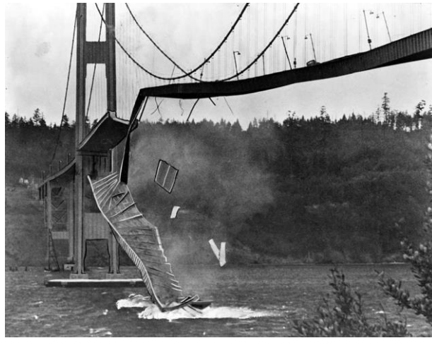
Figure 1. 11. Collapse of the Tacoma Narrows Bridge (1940)
