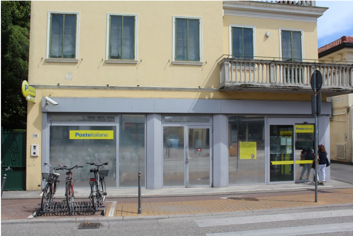
Figure 1 UP PD 7 - External façade
