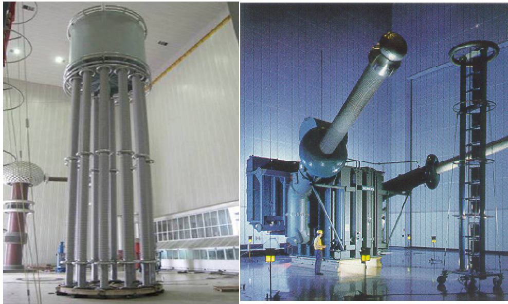
Figura 2.24 Smoothing reactor isolati in aria o in olio
