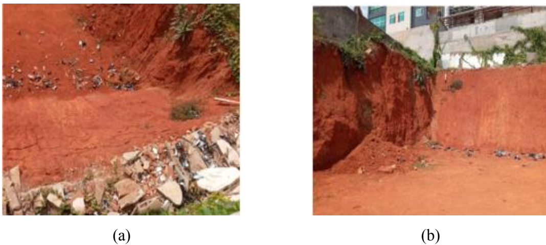
Figure 3.3. View of the project (a) Plan view (b) Side and front view
