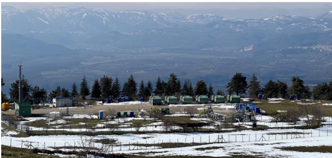
Figure 6: reinjection well Costa Molina 2, Montemurro (PZ)
