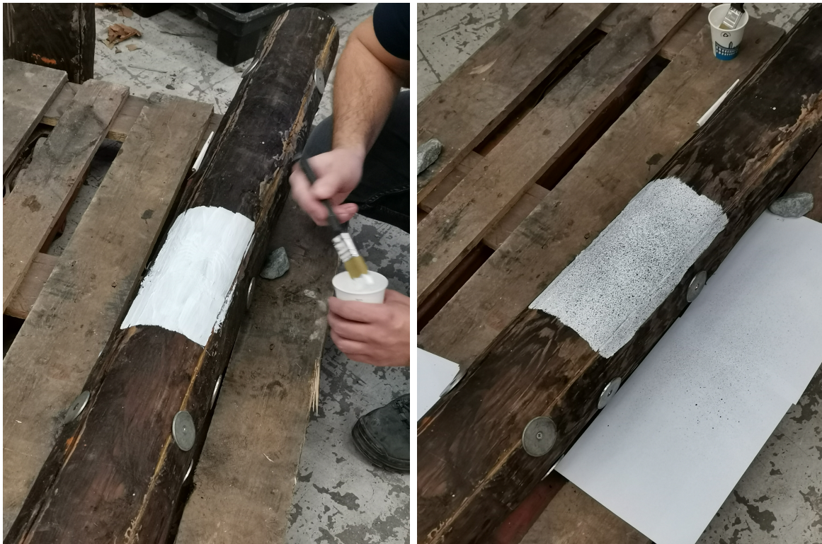
Figure 5.3.5: Painting of the pile surface;
