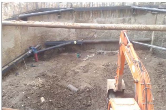
Figure 4.21: View of the work after the execution of CSM
