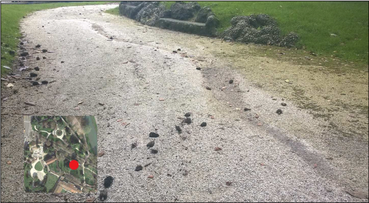
Figure 3.10 Rills in the soil due to a huge quantity of water.
