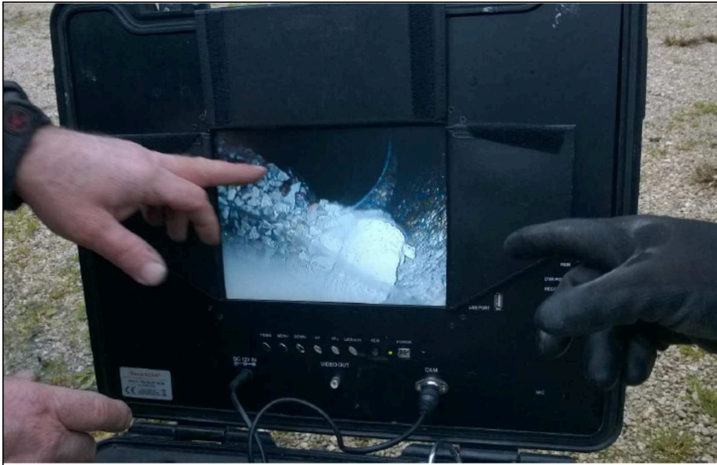
Figure 3.4 Visual inspection of a conduit that results interrupted.
