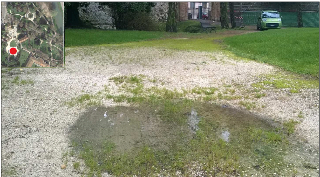
Figure 3.7 Area of stagnation of rainfall water
