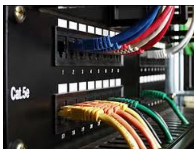
Figura 2.35: Patch panel per cavi in rame
