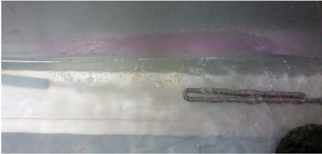
Figure 5.10: Inside of the tank on function and detail of its color. The pink is a bit enhanced to let it see in a better way.
