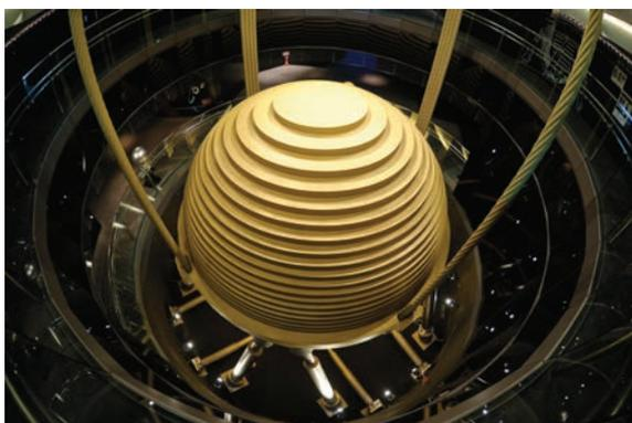
Figura 6.2: Smorzatore a massa accordata, TMD (Tuned Mass Damper).
