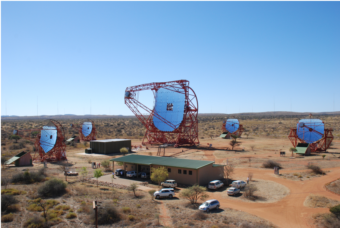
Figure 2.10: View of the full H.E.S.S. array with the four 12 m telescopes and the 28 m H.E.S.S. II telescope in Namibia (image credit: H.E.S.S. Collaboration, Clementina Medina)
