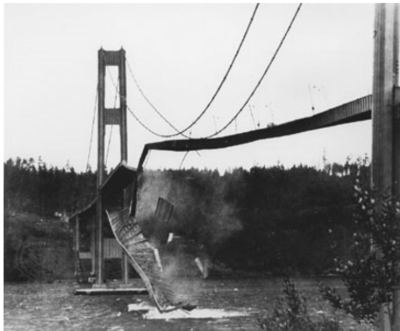
Figure 1.7. Collapse of the original Tacoma Narrows Bridge in 1940(Choudhury & Hasnat, 2015).
