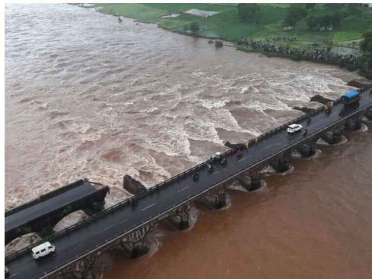
Figure 1.2. Bridge collapse due to flooding at Mahad over Savitri River of India (Limaye & Pujari, 2020).
