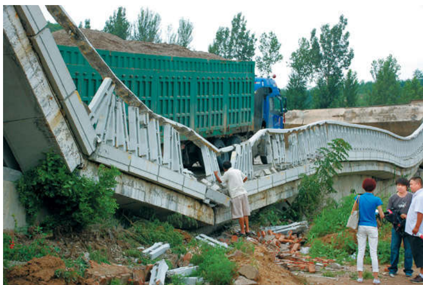
Figure 1.9. Bridge collapse due to an overloaded truck(Garg et al., 2020).
