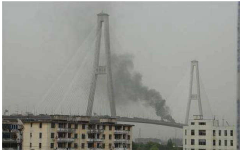
Figure 1.11. Close up of Xupu bridge fire, May 3, 2011 (Liu et al., 2012).
