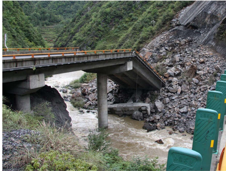
Figure 1.5. Collapse of a bridge due to landslide(Lin et al., 2012).
