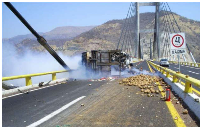
Figure 1.10. Truck overturned on Mezcala Bridge (Garlock et al., 2012).
