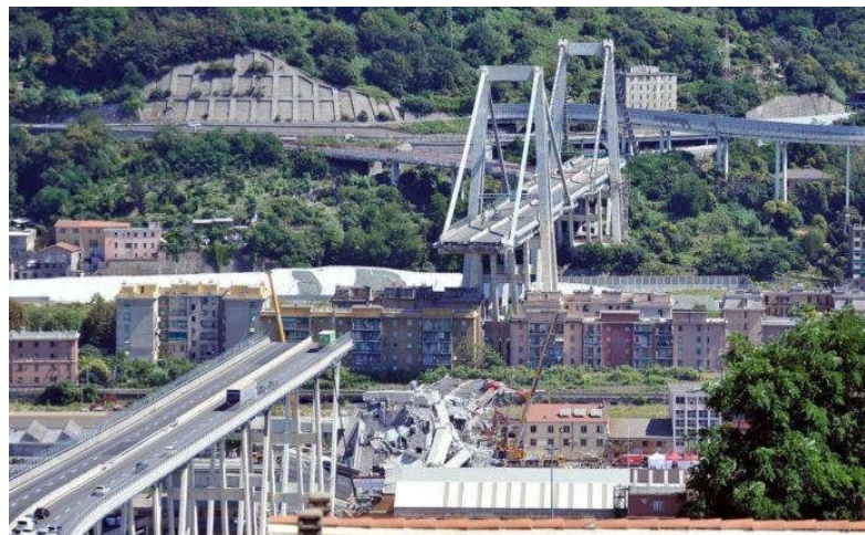
Figure 1.14. Collapse of Morandi Bridge Genova(De Matteis et al., 2019).
