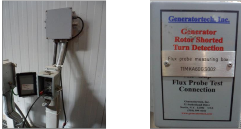
Figure.3.10: The external connection of the flux probe.
