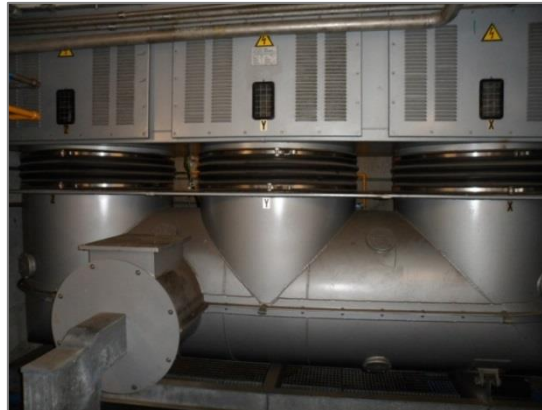
Figure.5.14: Neutral grounding of the synchronous generator.
