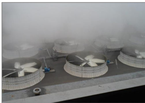
Figure.1.4: Eight cooling towers, forced ventilation.
