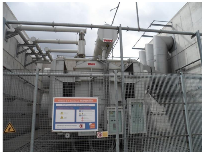
Figure.1.8: Step-up transformer.
