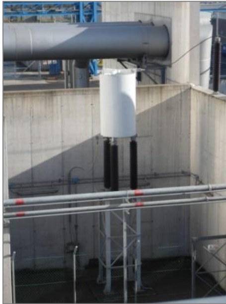
Figure.5.16: Step-up transformer neutral grounding reactor.
