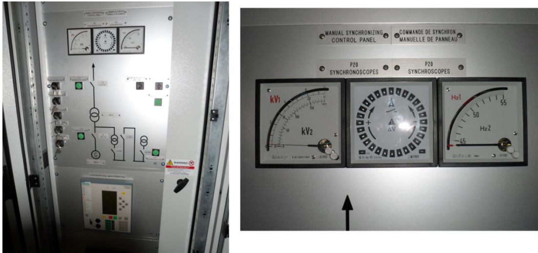
Figure.2.8: The synchronism cubicle.
