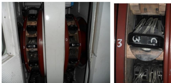
Figure.2.13: The excitation system (collector and the rings), focus of a brush.
