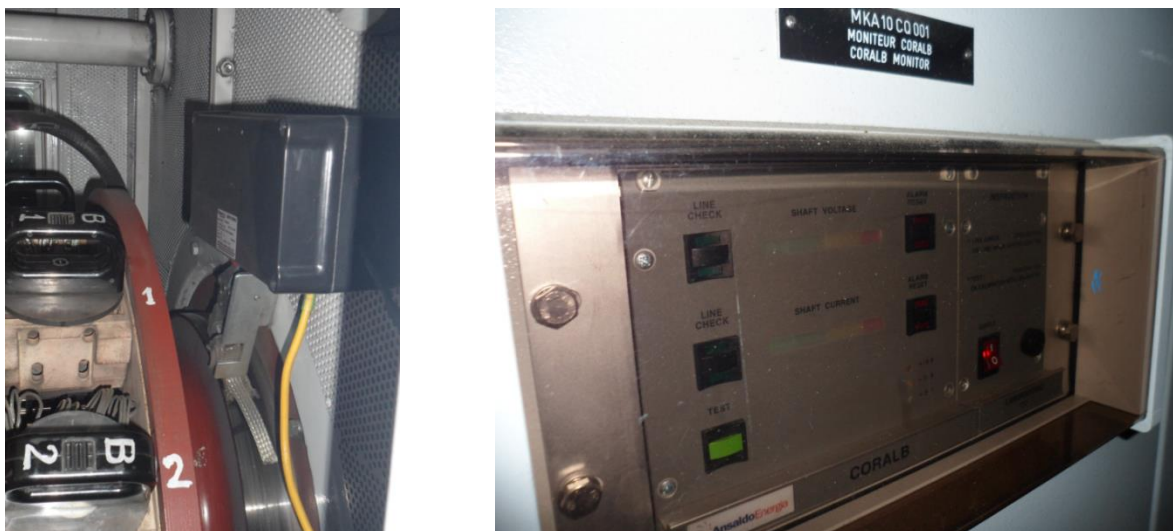
Figure.3.14: The crawling contact and the shaft supervisory cubicle with shaft voltage and current meters.
