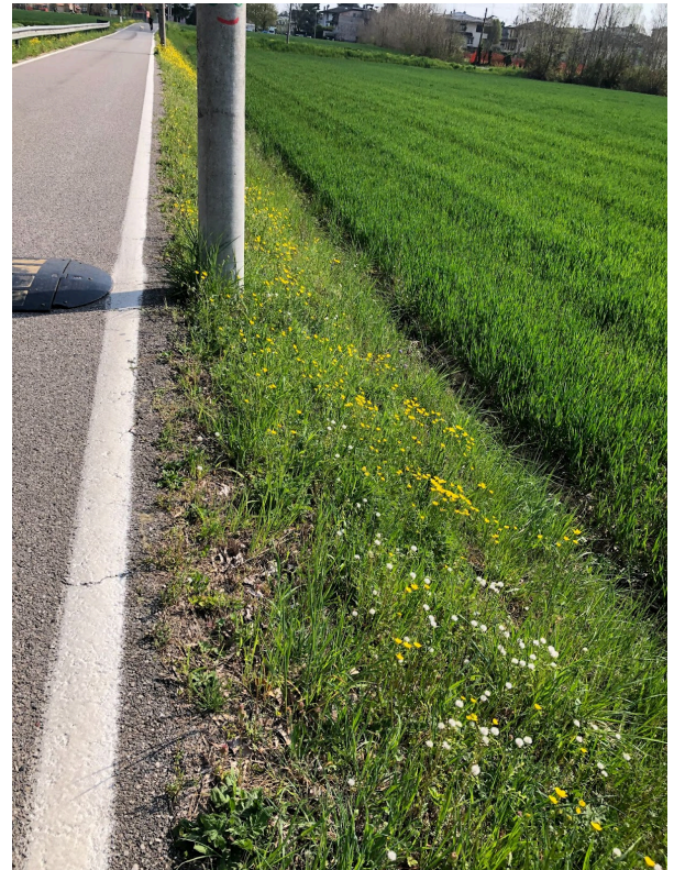
Fig. 1.10: Via Monte Pertica and the drop between the road and the ditch next to the field.
