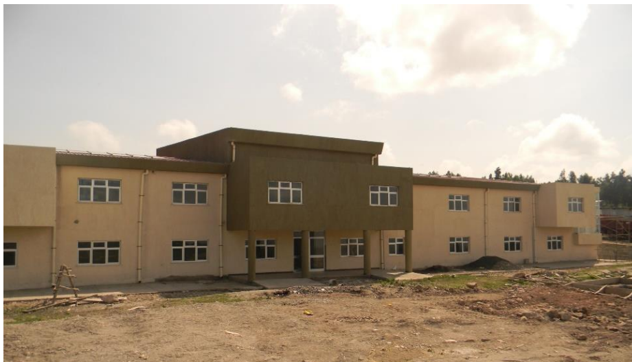
Picture 1 View of the southern facade of ISPEMA Center
