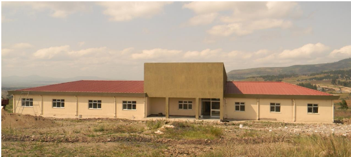
Picture 2 View of the northern facade of the building
