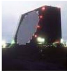
Cobra Dane (USA) detection limit: ≈ 5 cm at 1000 km
