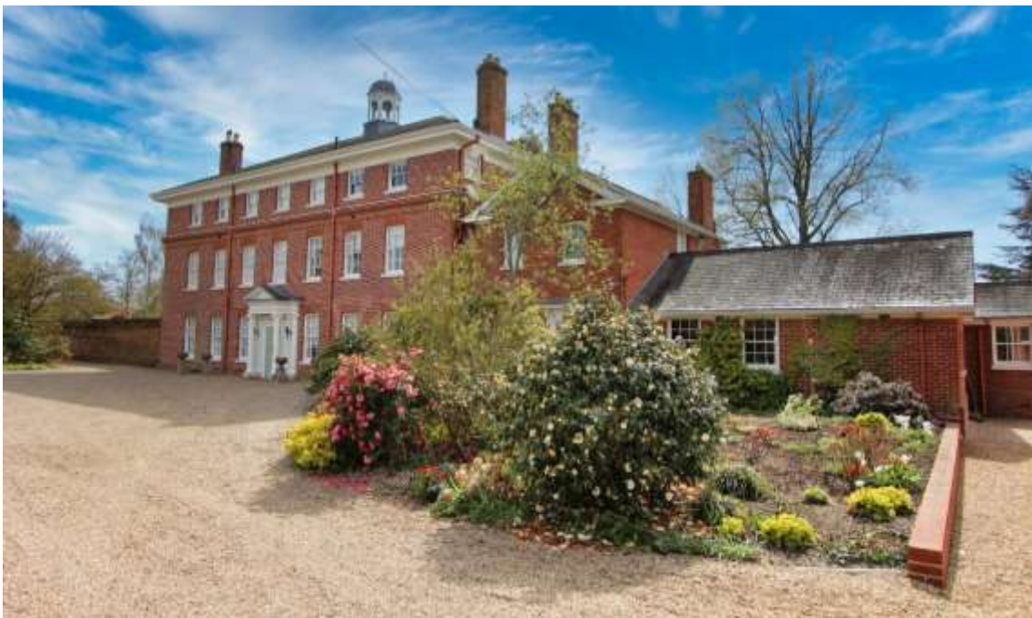
Fig. 28 West Lodge, oggi denominata Stour House.
