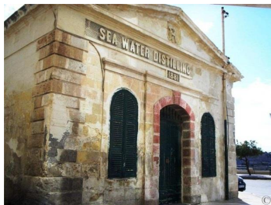
Figure 1.3: remains of the first desalination plant in Tigne (Malta)
