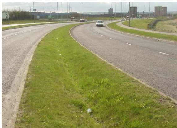
Fig. 5.9. Fosso d'infiltrazione (Fonte: Pittner C., Allerton G. 2010. Suds for roads. Scots - Suds Working Party – WSP. Scotland)
