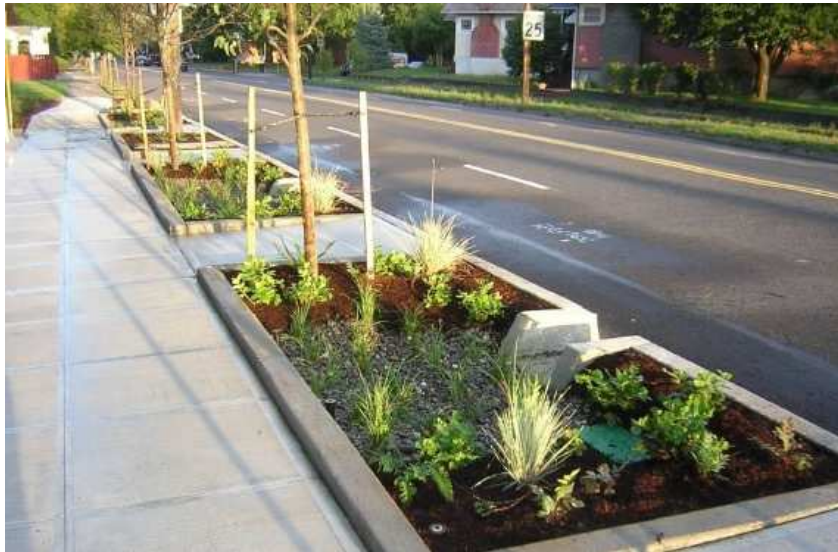
Fig. 5.28 Bioretention (Fonte: Pittner C., Allerton G. 2010. Suds for roads. Scots - Suds Working Party – WSP. Scotland)
