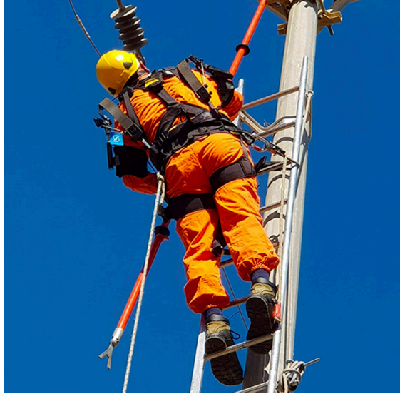
Figure 4.1: Skelex and Enel project to support workers in maintaining the electricity grid [38].
