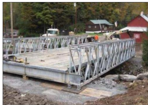
Figure 1.2. Panelized truss temporary bridge with two trusses on each side of roadway ( fdotwww.blob.core.windows.net )
