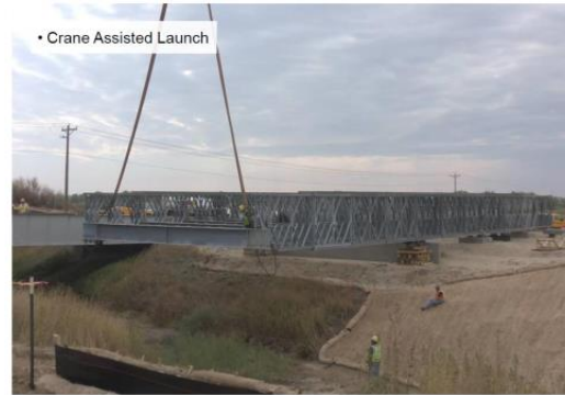
Figure 1.45. Crane assisted launching process ( Index @ Wwww.Lindependant.Fr, n.d. )
