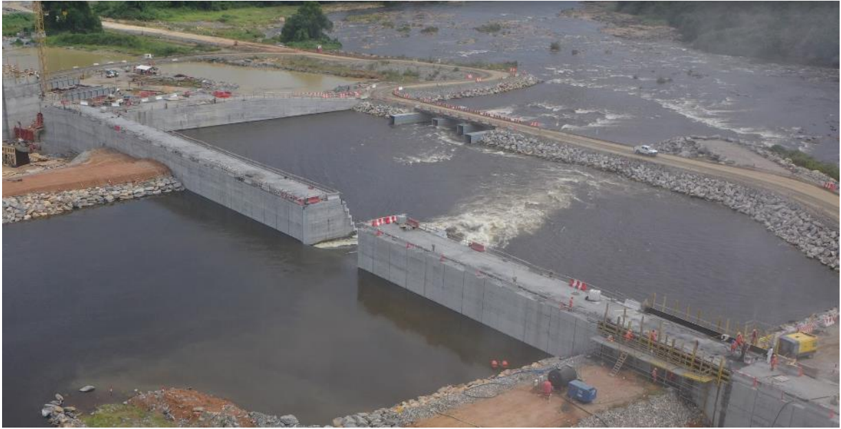
Figure 3.4. Side view of the Nachtigal Hydropower site
