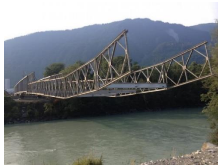
Figure 1.3. Installation of panelized truss with launching nose(www.maybeybridge.com)
