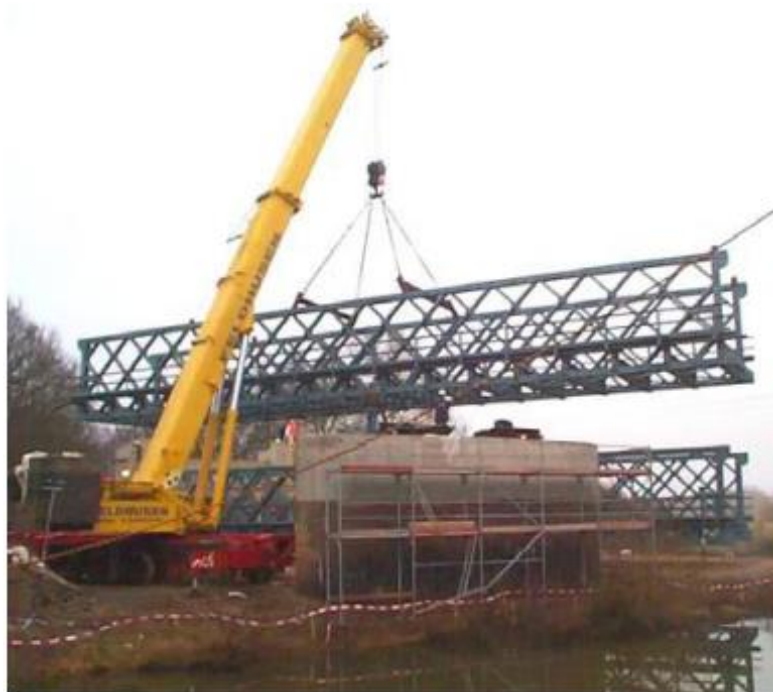
Figure 1.43. Bridge lifted in by a mobile crane( Index @ Wwww.Estrepublikain.Fr, n.d. )
