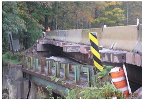
Figure 1.5. Steel Girder temporary bridge (fdotwww.blob.core.windows.net)
