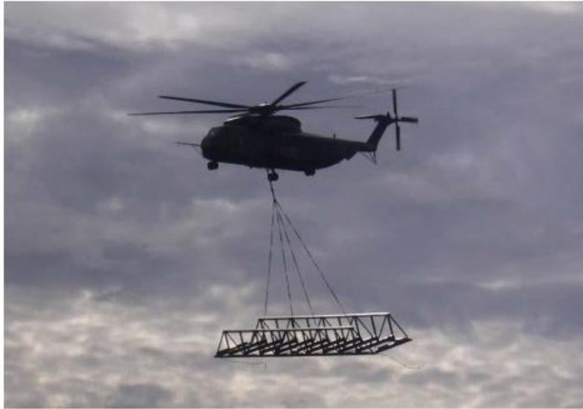
Figure 1.44. Bridge lifted in by helicopteter ( Index @ Wwww.Lindependant.Fr, n.d. )
