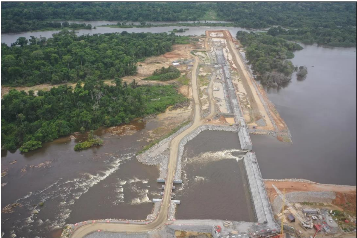
Figure 3.5. Aerial view of the Nachtigal Hydropower site
