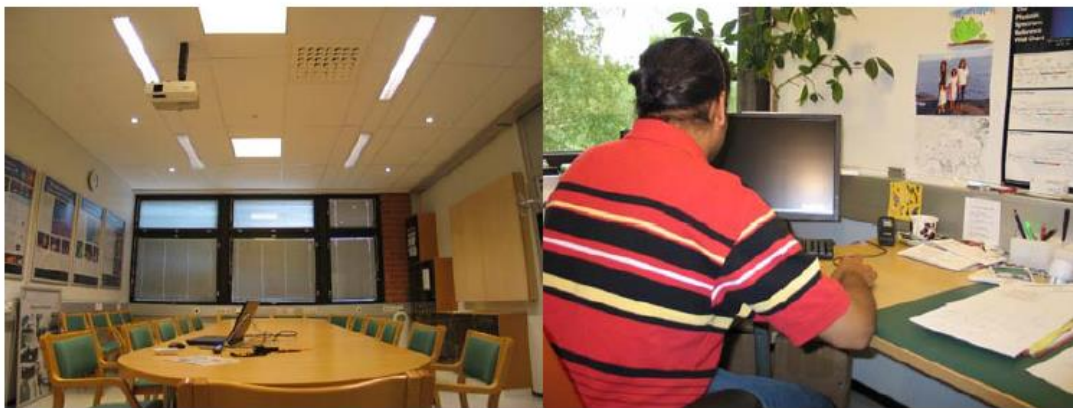
Fig. 2.4 Examples of luminaires and windows that can induce visual discomfort
