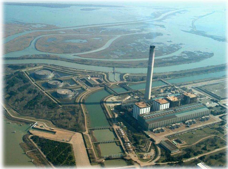
Figure 15: Enel power plant in Polesine Camerini” located in Porto Tolle, Rovigo, Italy.
