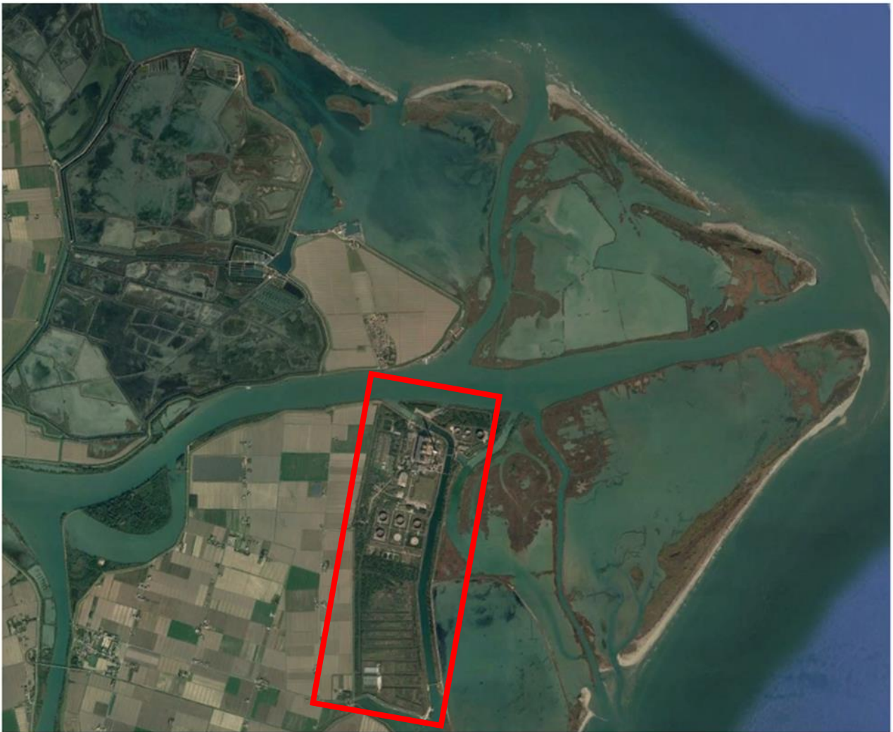
Figure 16: Location of the ex- power plant that is built on a river delta (Georicerche, 2024).
